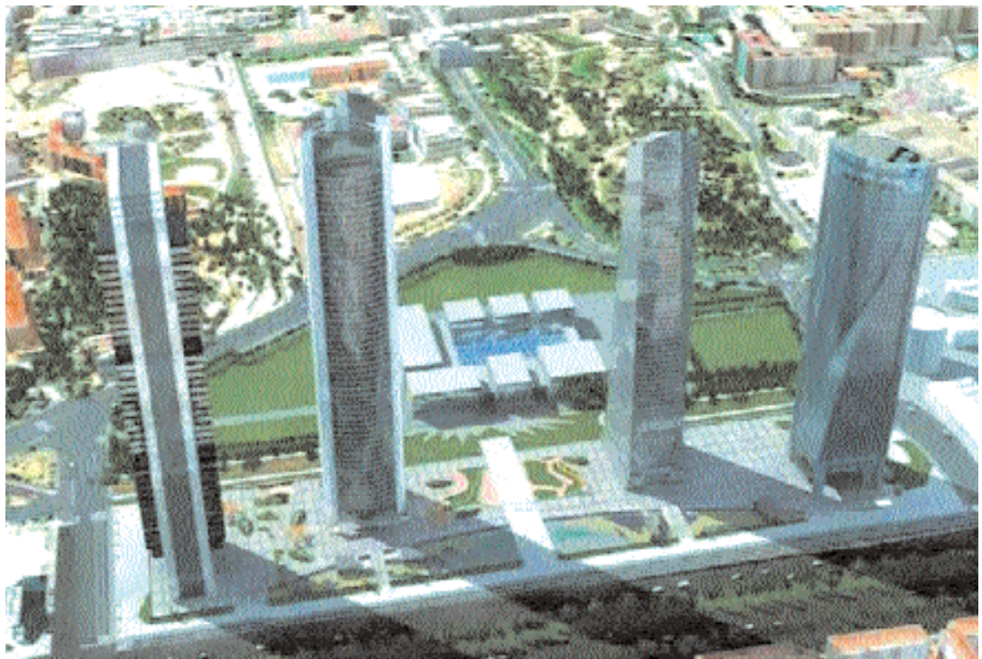
Il complesso CTBA "Cuatro Torres Business Area", a Madrid
